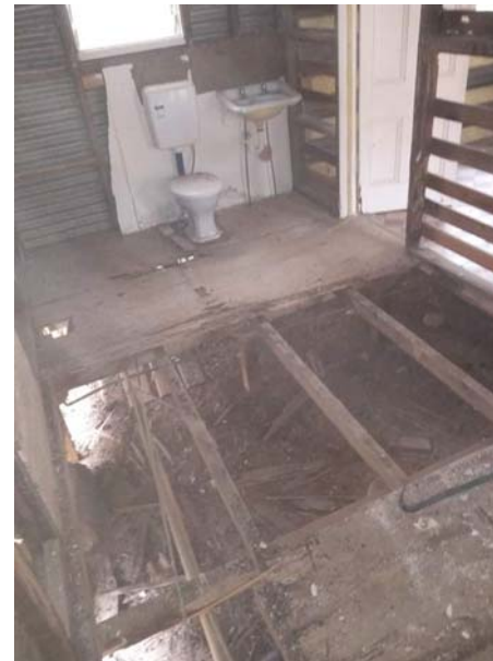
Before restoration work began in the hut
